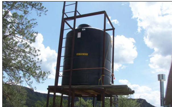
New Water Tank at Jenkins Cabin
