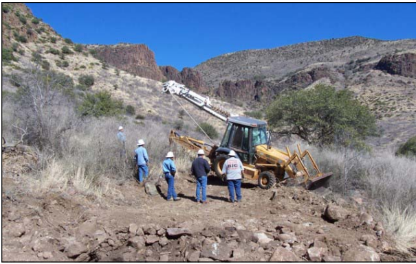
Power Line at Circle H
